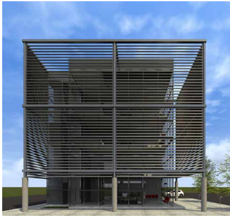
Perth Data Center, 2015
